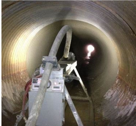
Picture 4: Lining machine applying.
