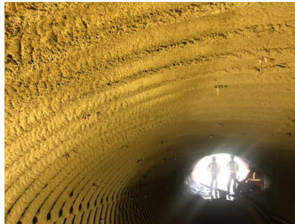
Figure 10: Pipe after first pass
