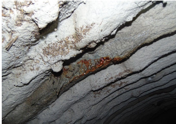
Figure 11: Culvert's Condition a Year After Liner Installation
