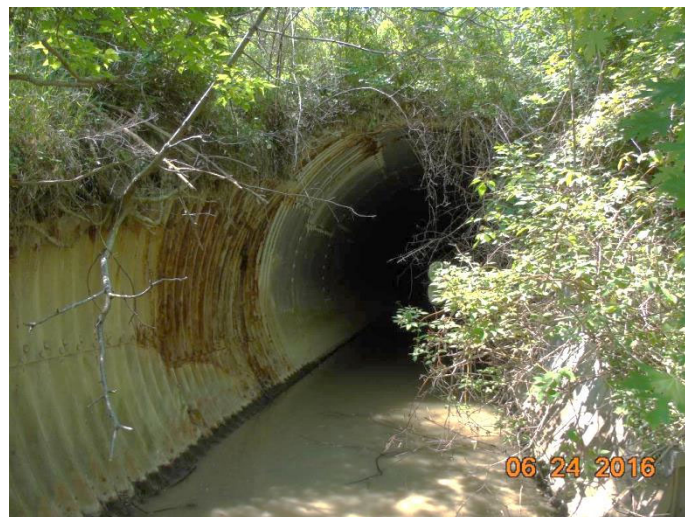
Figure 7: Pipe Corrosion at Entrance
